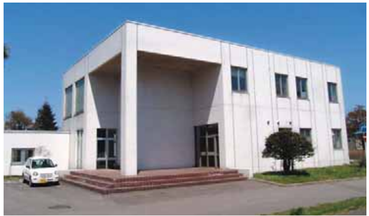
▲ 福利施設 Welfare Facilities
